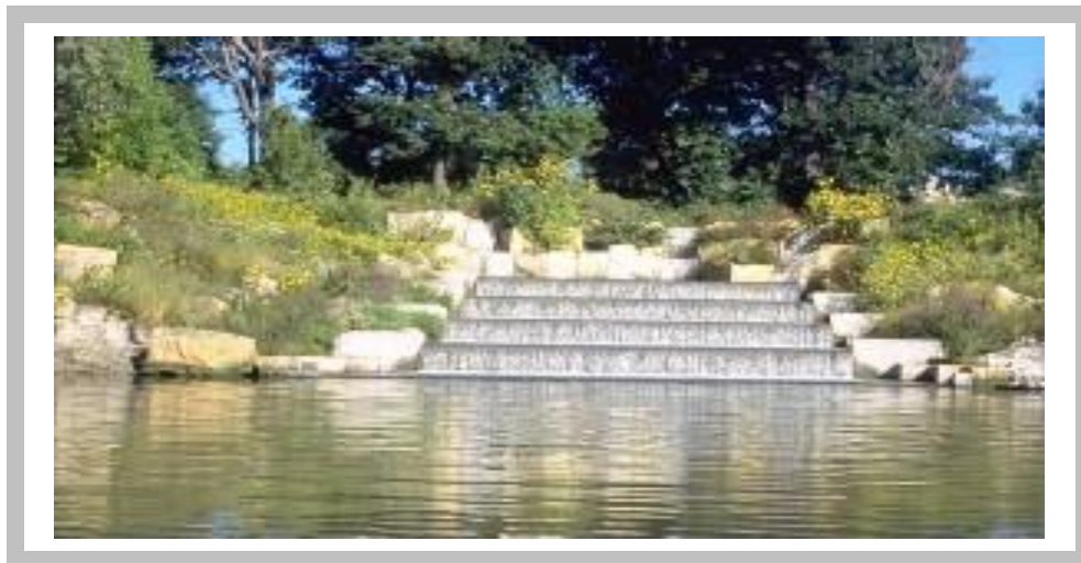
Figure 5-5 - Side-Stream Aeration Facility
