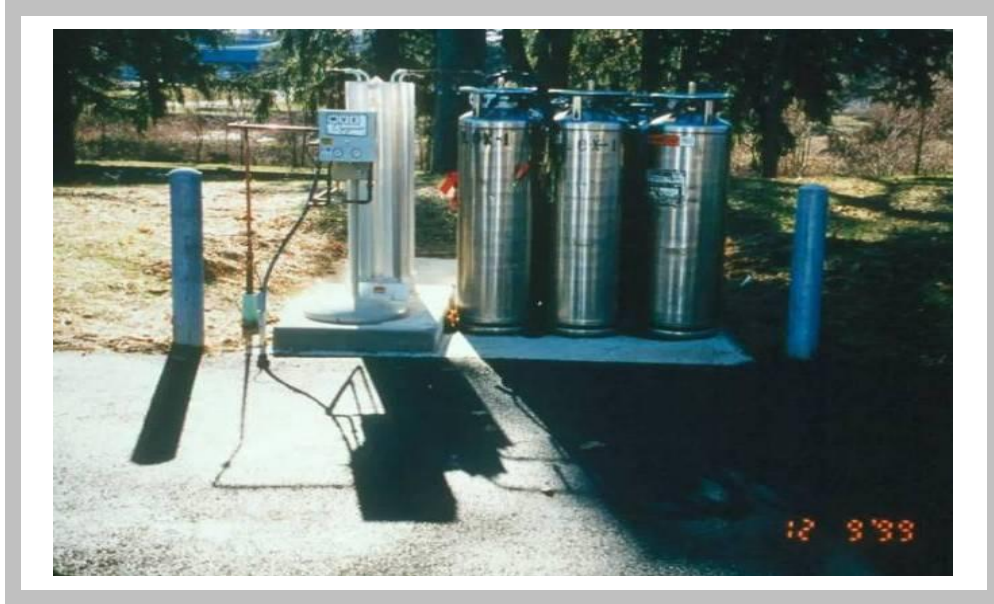
Figure 5-3 - Low Head Oxygenators
