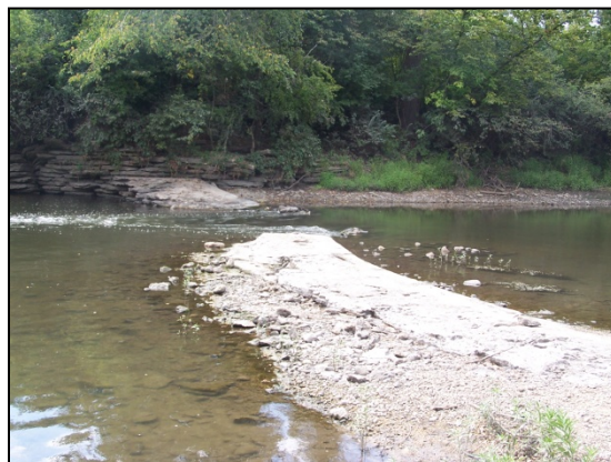
Plate No. 2. Remnants of the McDowell Grove dam used to form a riffle after its removal in 2008. The riffle and former structures remain in place.
