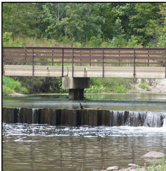
Plate No. 3. Temporary cofferdam constructed upstream from the former McDowell Grove Dam in 2008. The cofferdam was removed in the fall of 2012, immediately after the 2012 survey.
