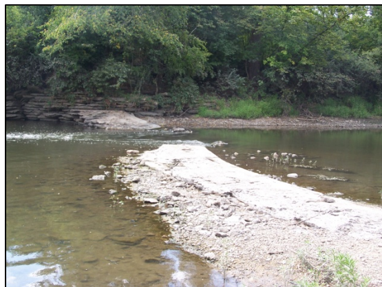
Plate 2. Remnants of the McDowell Grove dam used to form a riffle.
