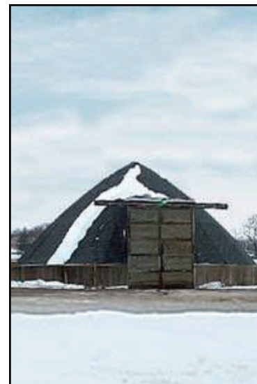
Salt dome used for storage.
